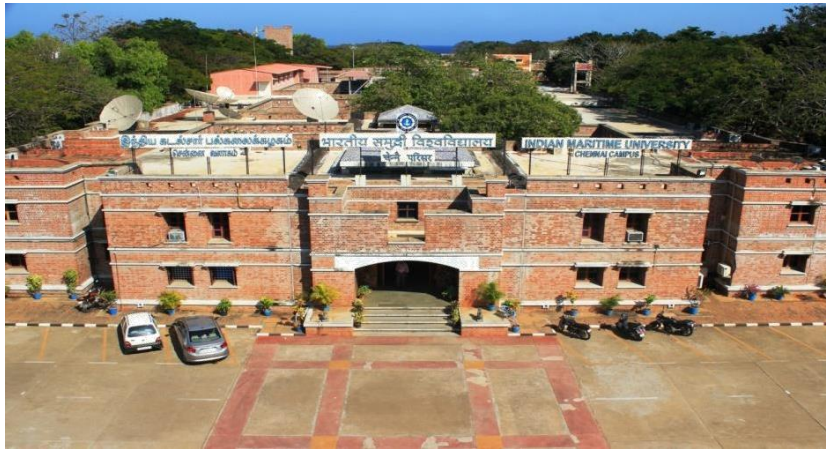
Aerial View of IMU, Chennai Campus
