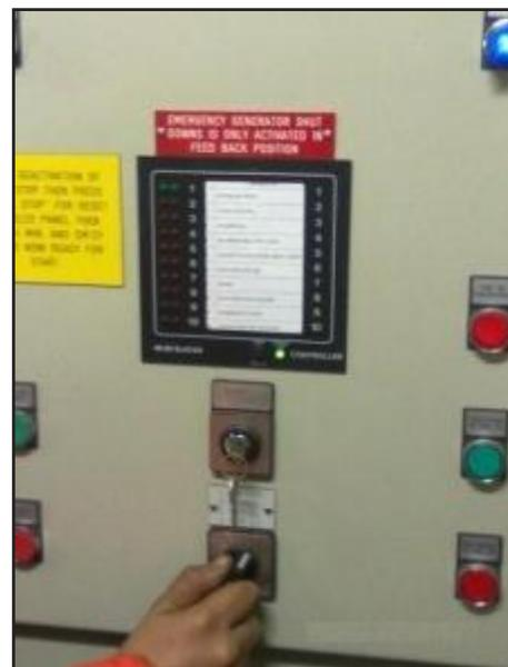
different marine diesel emergency generator set, it is extremely important to be completely familiarized and well trained to an extent that in case asked by any shore officials, the crew member should be able to demonstrate the same.
